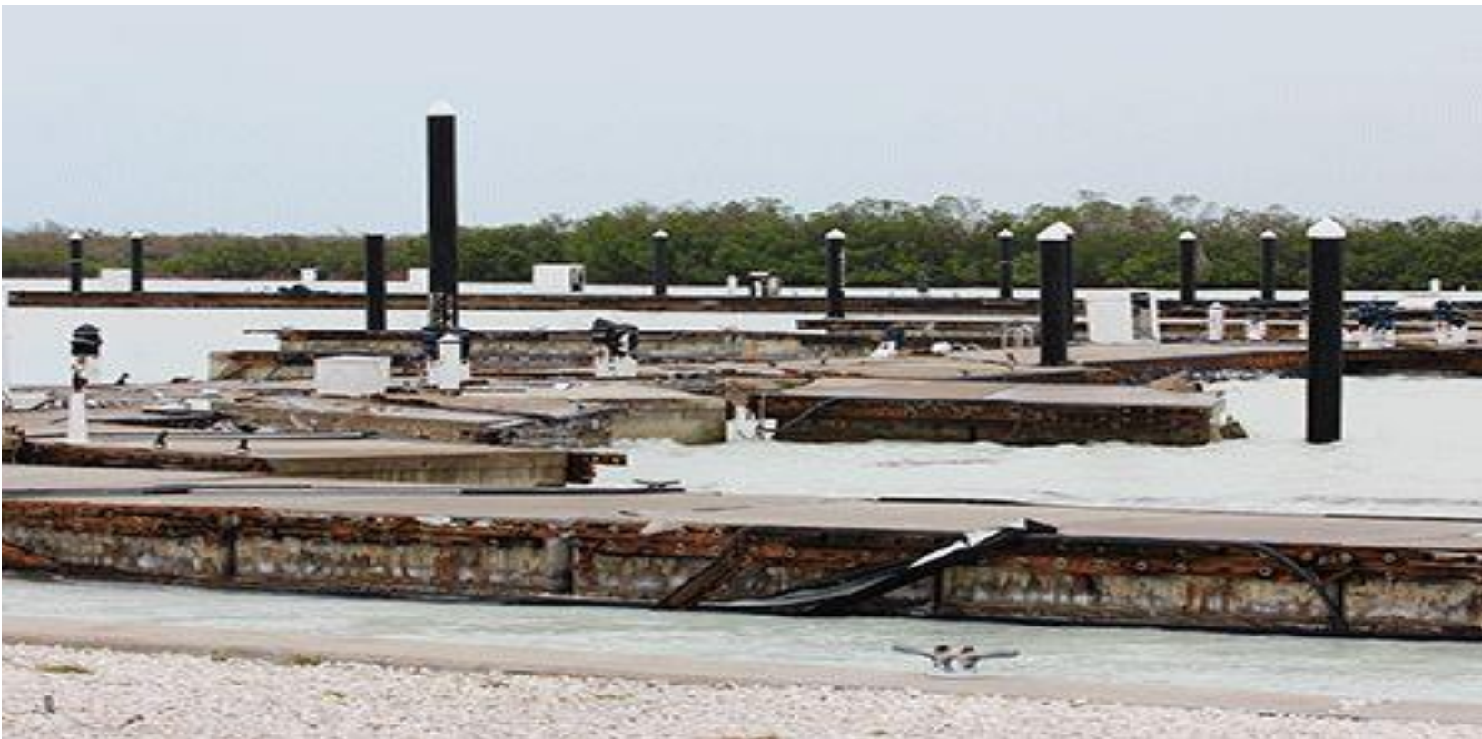
Destroyed concrete docks after Hurricane Irma in 2017
