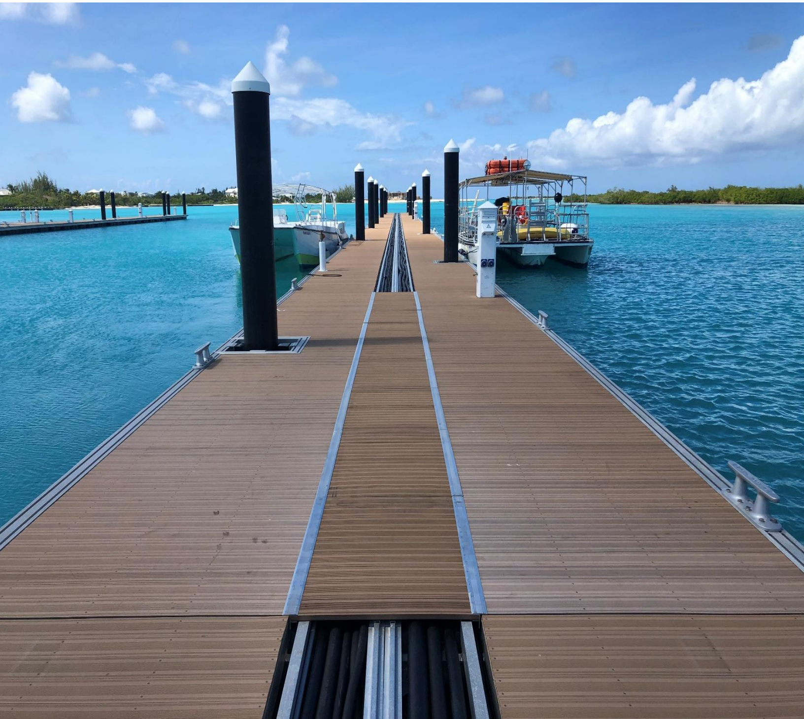
Large central utility trough makes installing and maintaining utilities fast and simple
