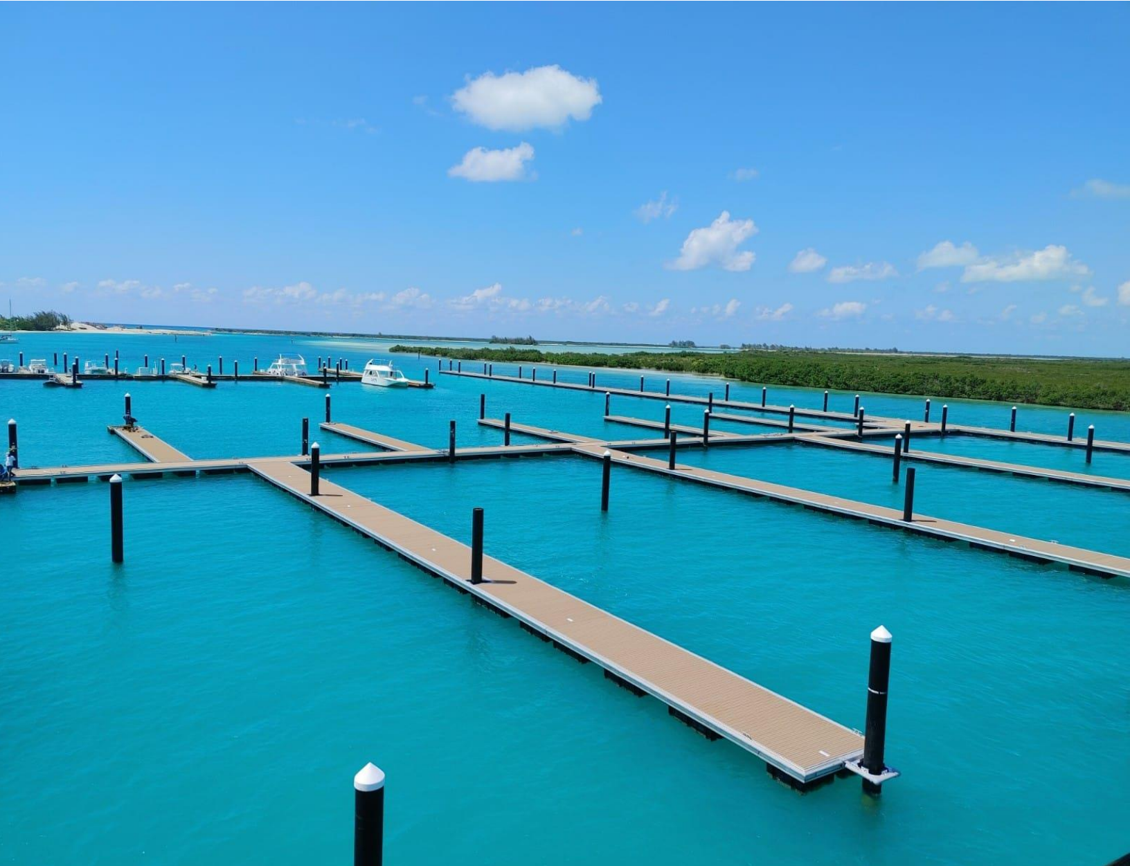
71 slips for mega-yachts up to 220 ft long, anchored with steel pipe piles
