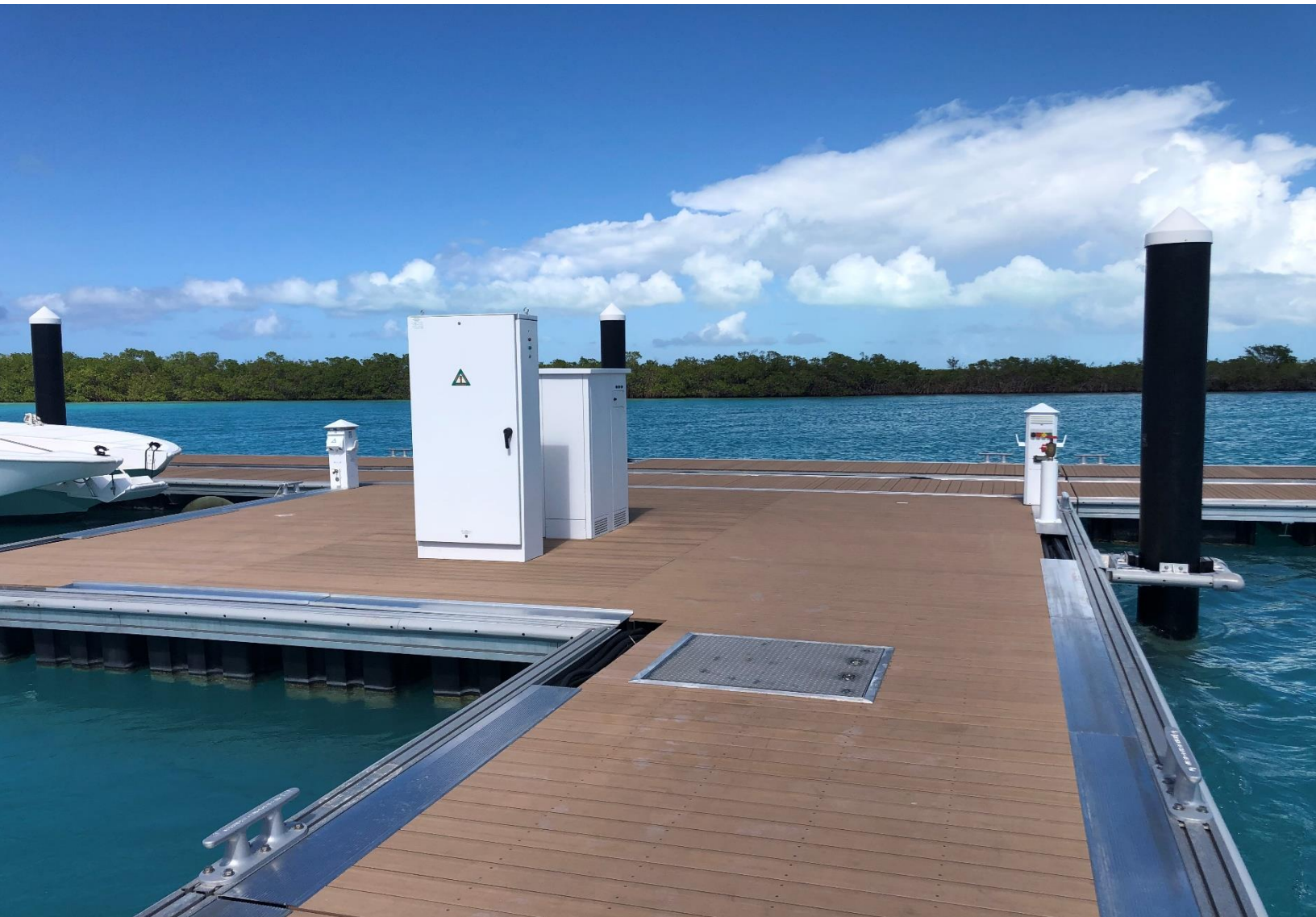
Built-in fuel hydrants, under cover, for hi-speed diesel delivery – no pumps on docks
