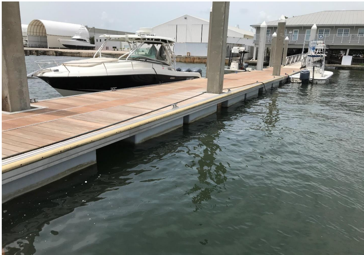
New Marina Technologies System D-260 aluminum docks with high-stability concrete floats
