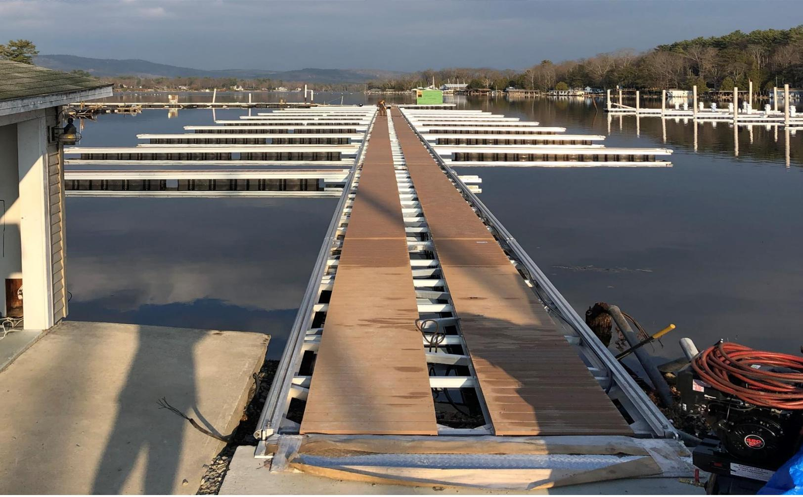
Dock and pile Installation is now completed, and utilities are being finalized. 10-inch PVC piles were used to anchor the docks, which will provide superior performance with minimal maintenance for decades, says Berry.
